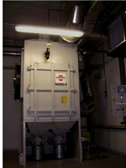
Decentralized filter with flameless pressure discharge
