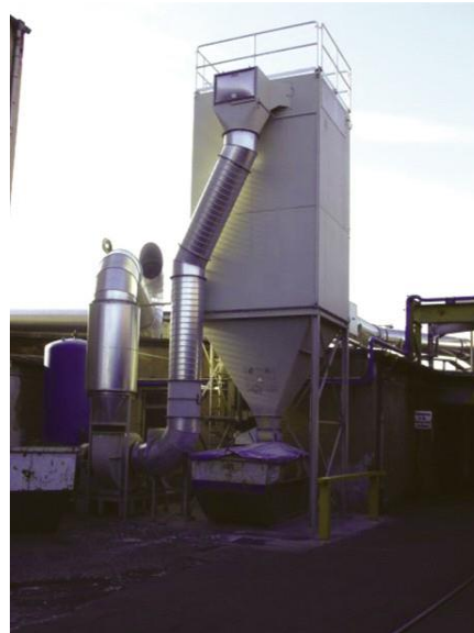
Centralized filter with constructive explosion protection
