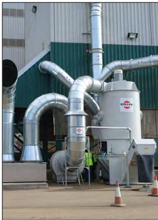
Wet scrubber VDN-AS with de-sludging device
